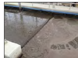
Transport baffles to reduce airlift trapping
