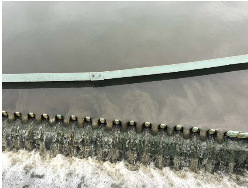
Figure 3-10 Observed Loss of Solids at Clarifier 6 During Stress Testing
