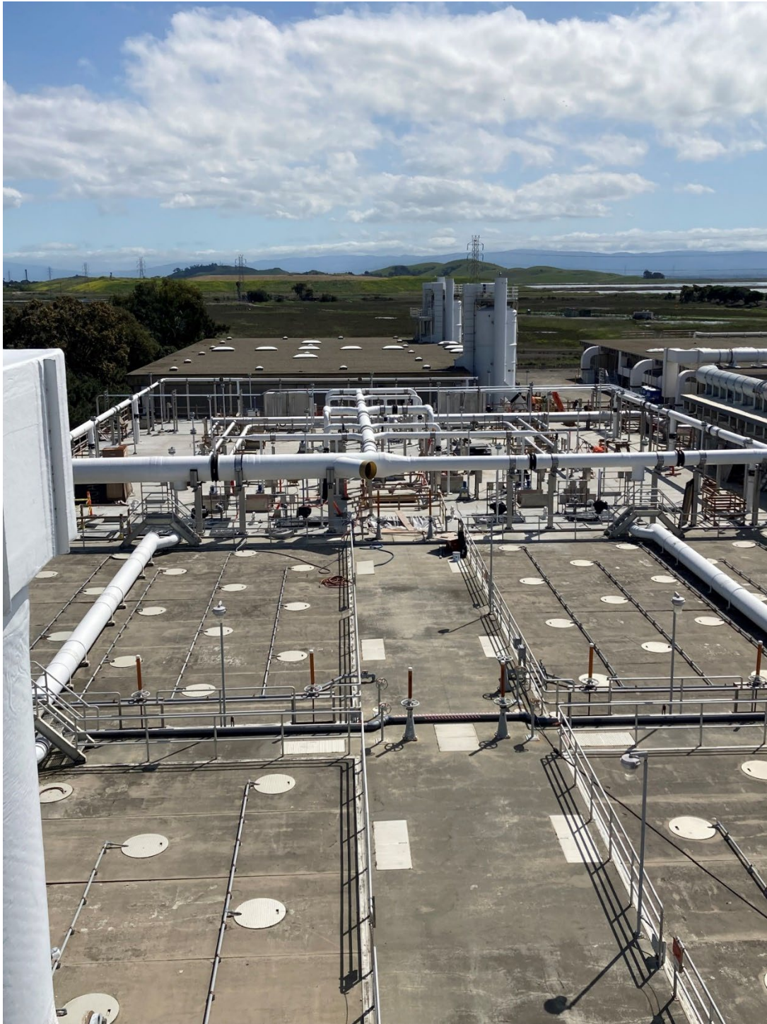
ETSU East Aeration Basin Construction
