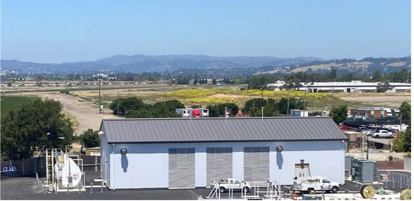
New Standby Power Building
