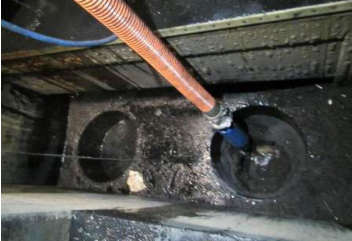
Figure 3 – View above the two force main inlets at CB1
