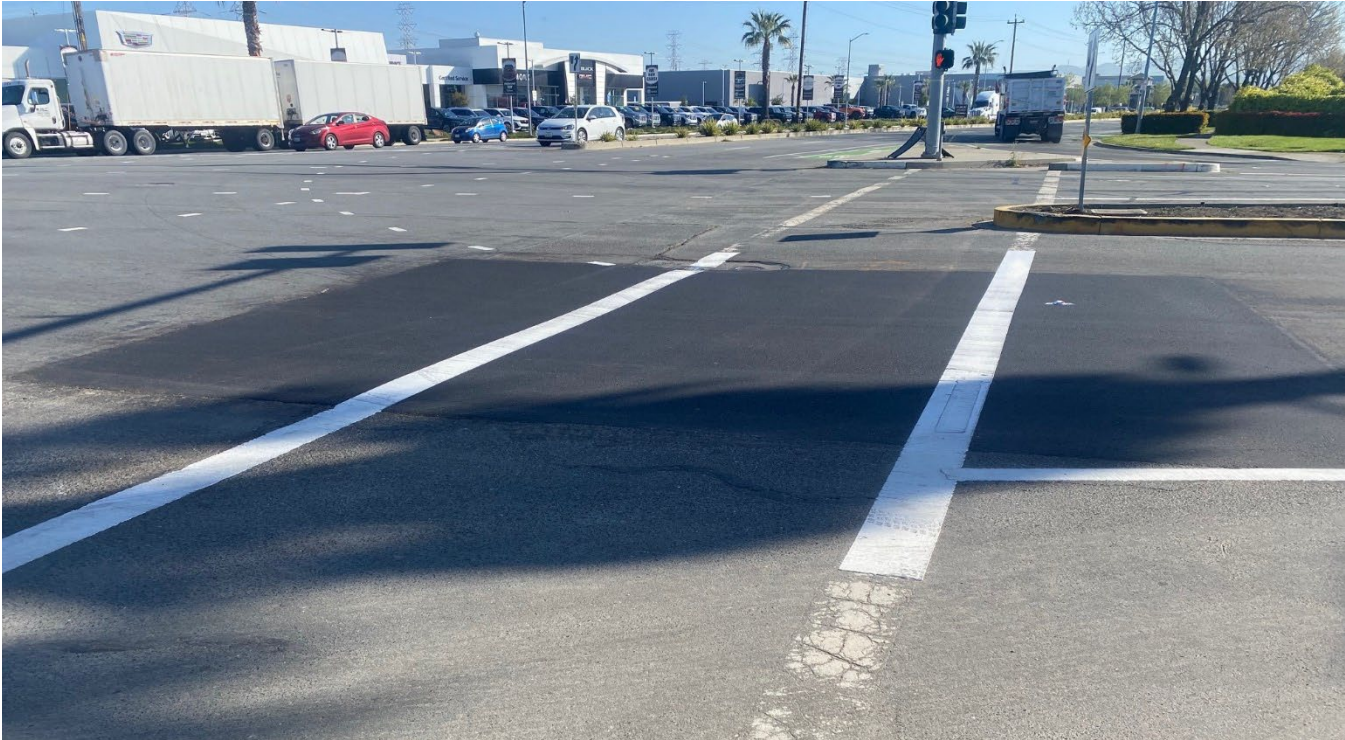
Figure 3 – Completed Repair of Intersection
