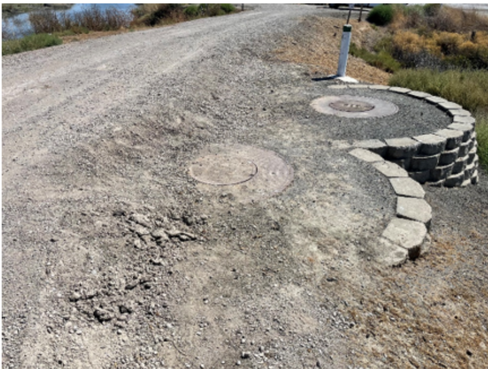
Figure 10 – Grading and Retaining Wall at Cushing Parkway No. 1 Access Manhole
