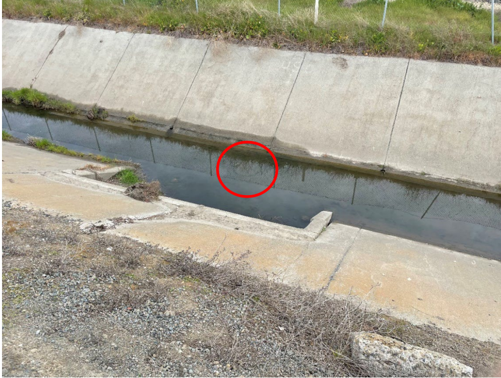
Figure 11 – Cargill Salt Fields South Manhole to be Abandoned
