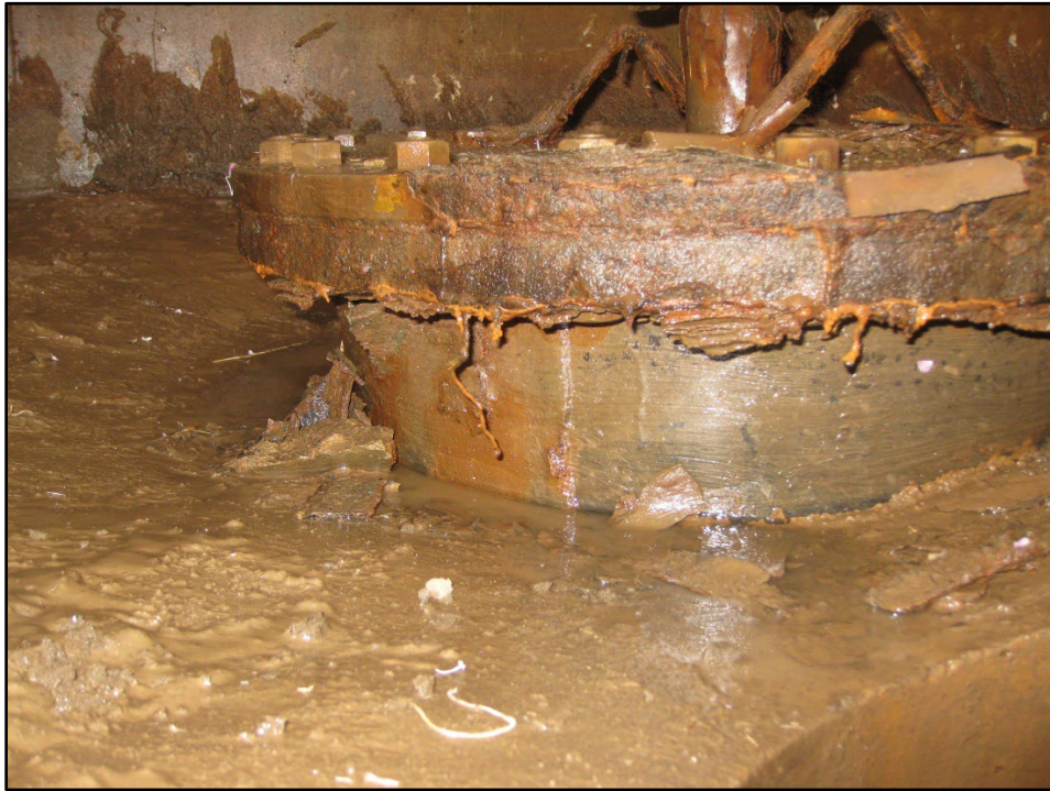
Figure 3 – Manway at Cargill Salt Fields North Access Manhole
