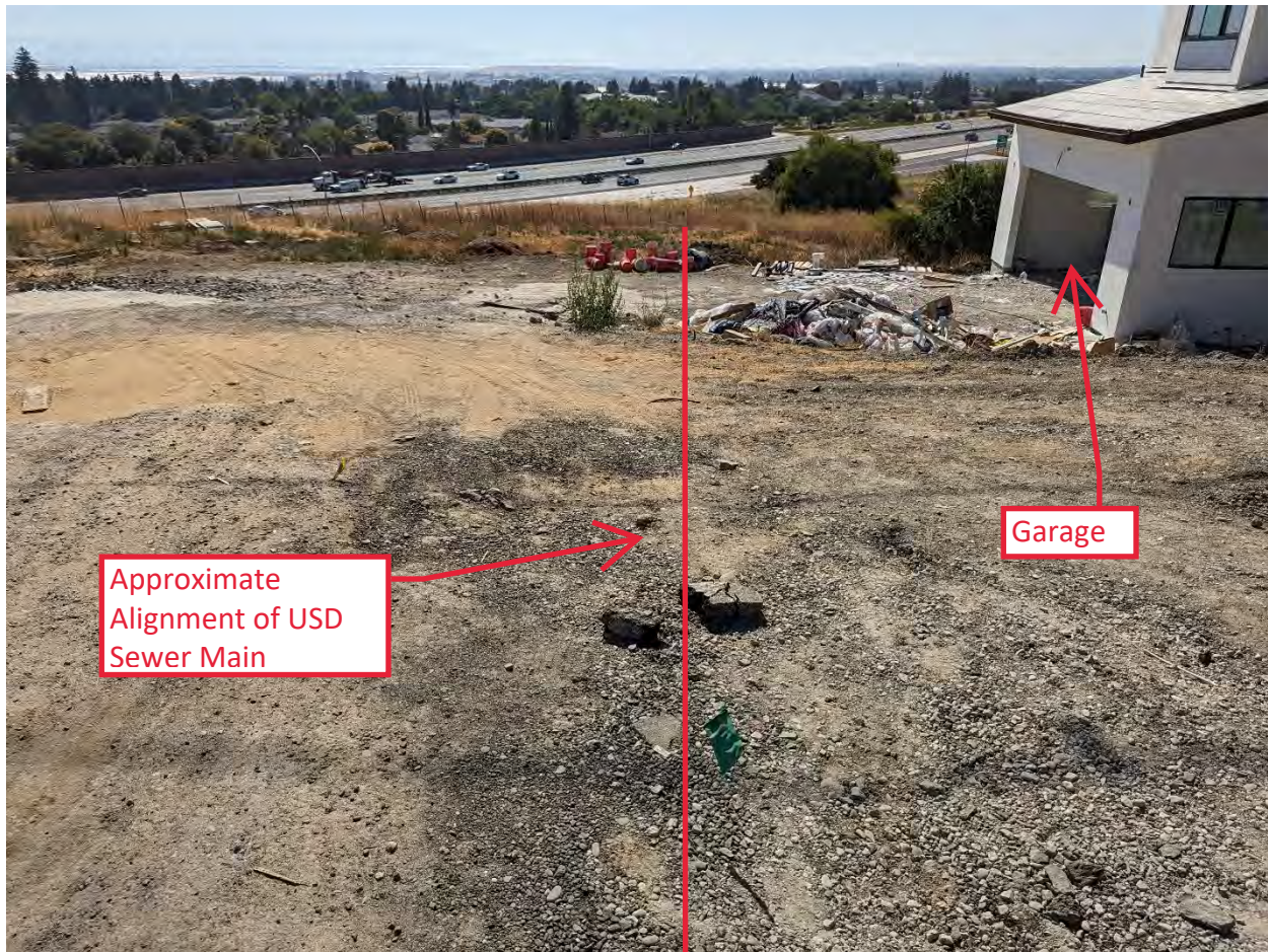
Figure 3 – Looking northwest down the slope of the property with Interstate 680 in the background
