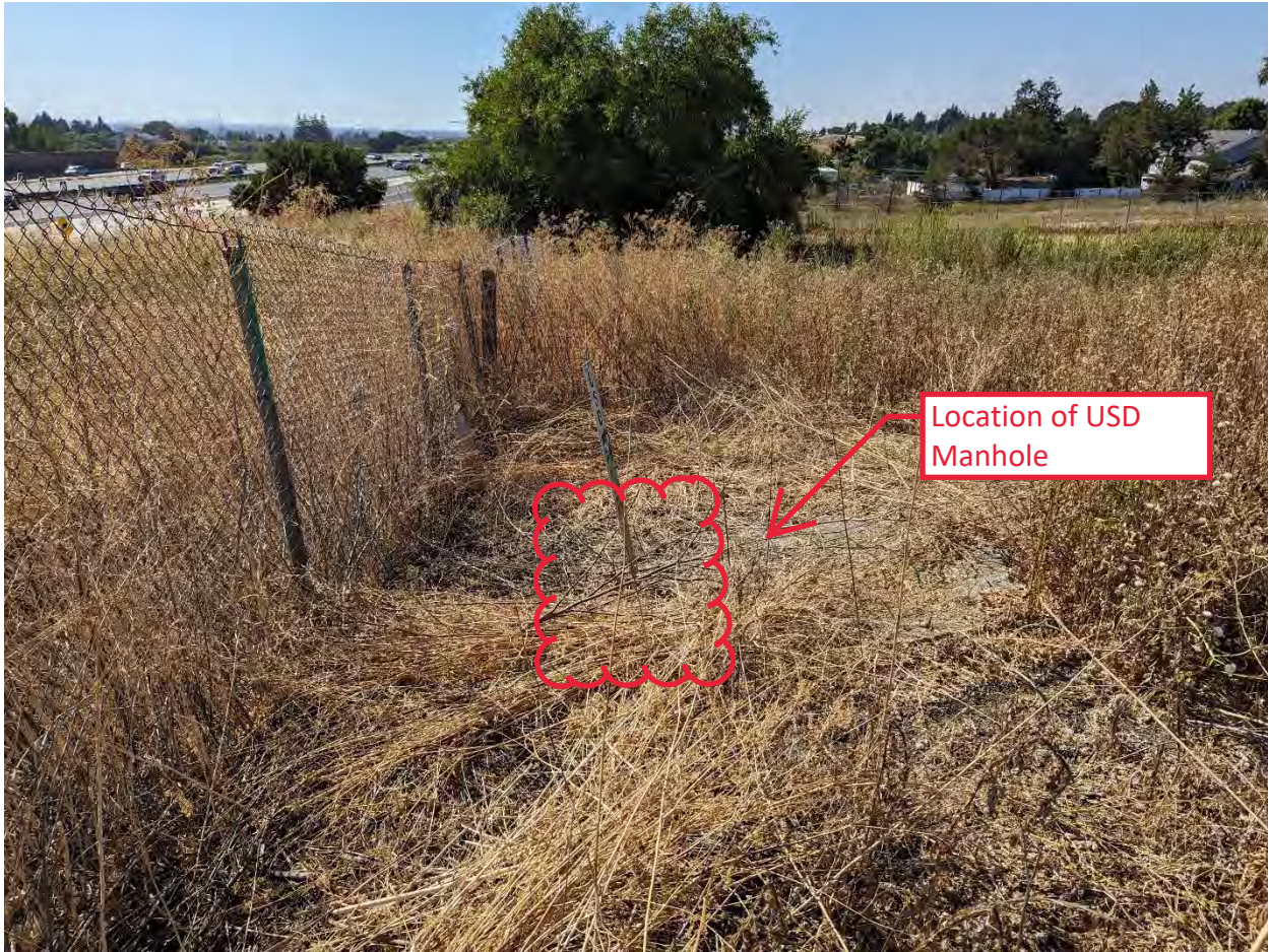
Figure 5 – Existing USD manhole located under the brush in the western corner of the parcel
