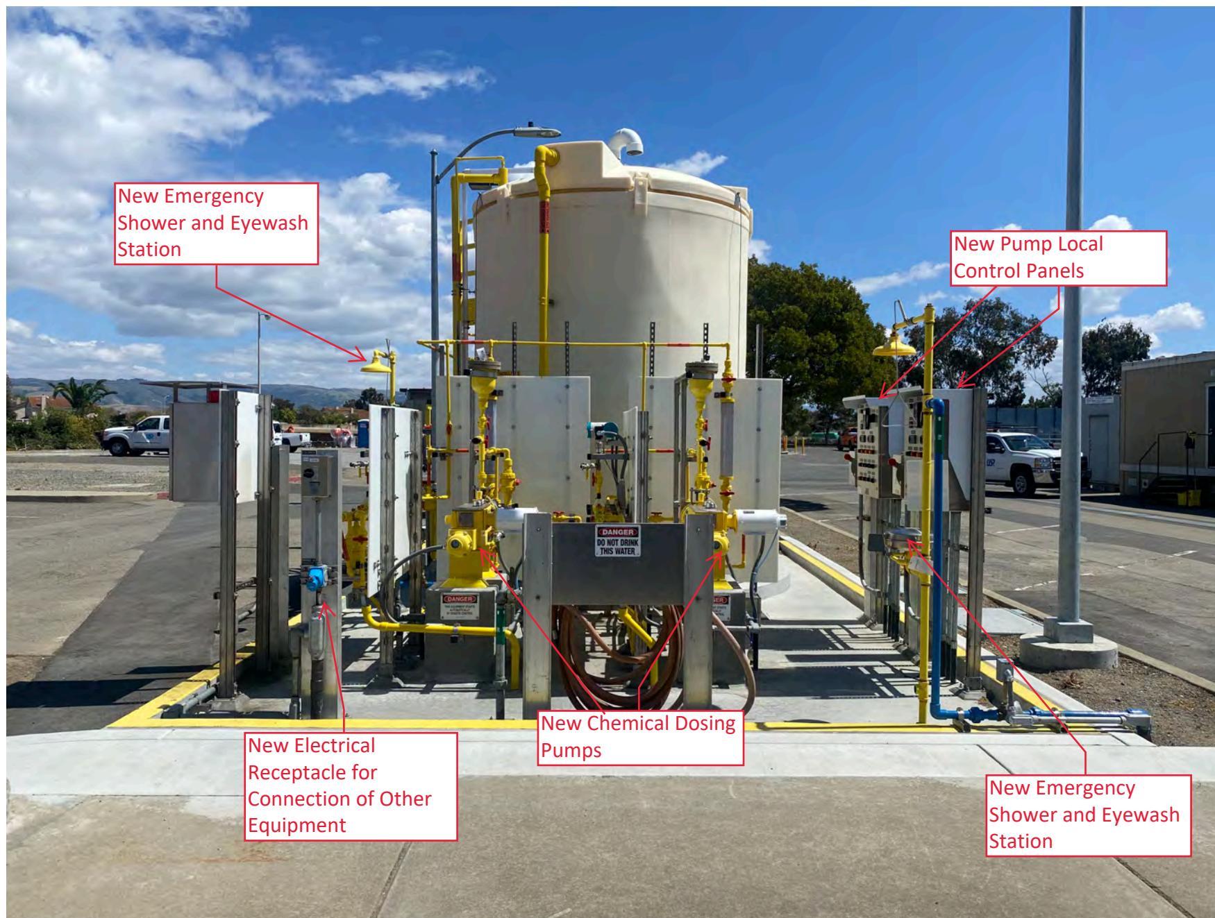
FIGURE 4 - New Calcium Thiosulfate Feed System Facility Looking West
