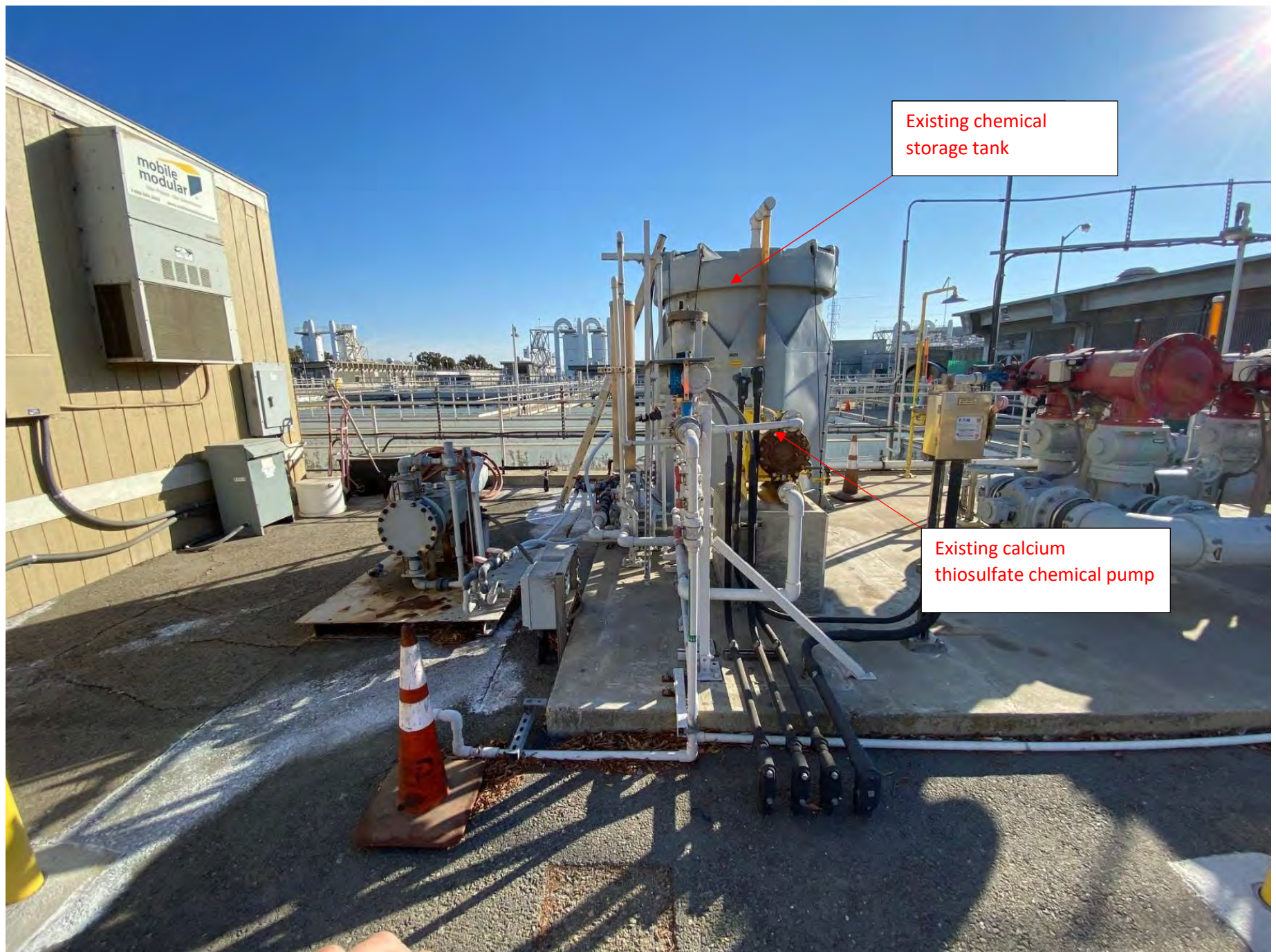
FIGURE 2 – Existing Calcium Thiosulfate Chemical Feed System
