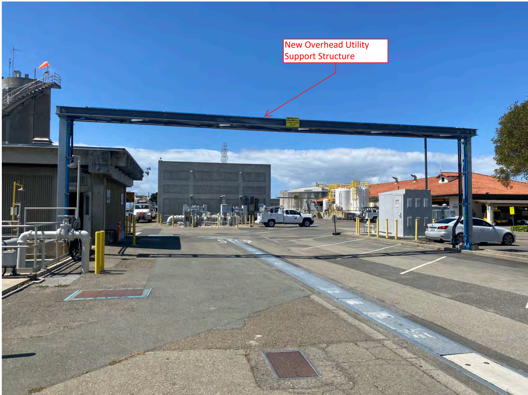
FIGURE 6 - Overhead Utility Support Structure
