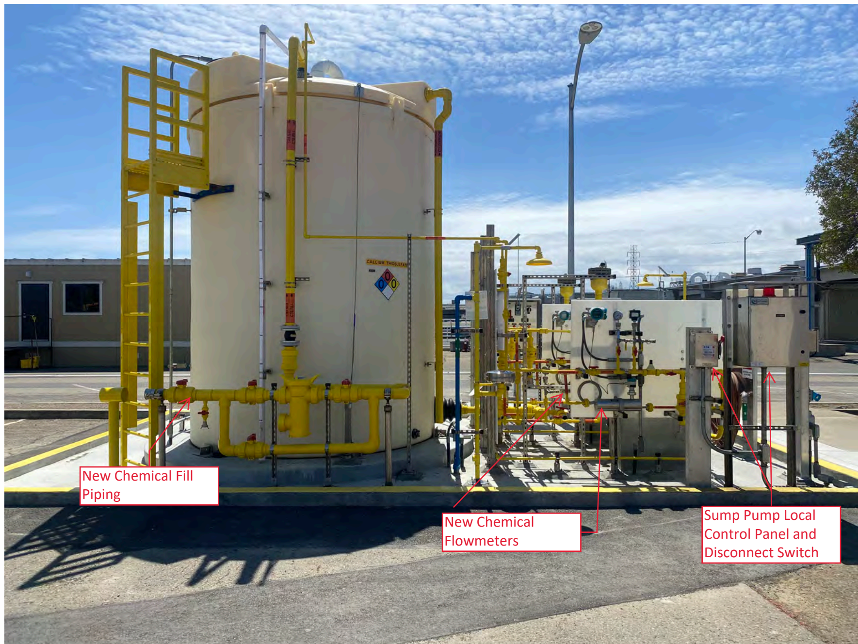
FIGURE 5 - New Calcium Thiosulfate Feed System Facility Looking South
