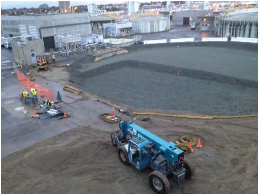
Installation of K-Rail and Safety Fencing Around Site Post-Demolition
