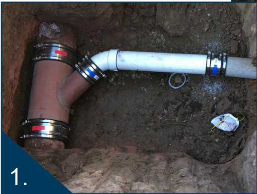
Photos of Open-Trench replacement of a lateral: (1) Connection of the lateral to USD’s main in the street; (2) Gravel dumped for bedding the pipe; (3) A properly bedded lateral – view from street to curb;
