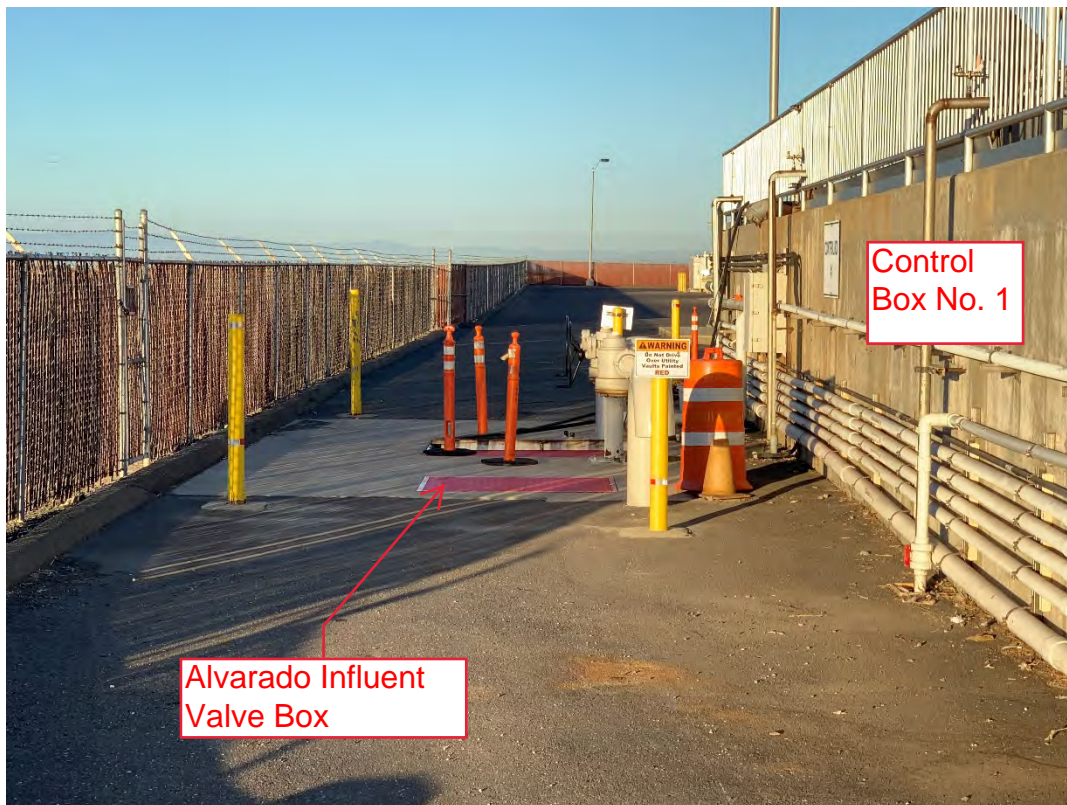
Figure 4 – Alvarado Influent Valve Box (Twin Force Mains and Valves Inside)
